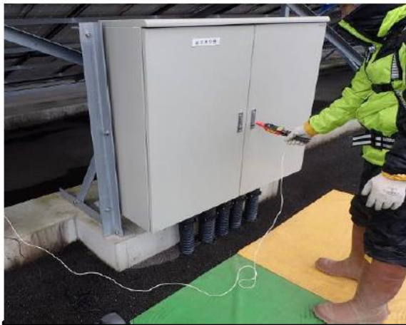
盤、盤架台の検電
